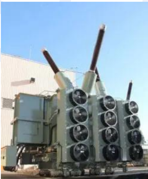
Fig (g): OFAF cooling of transformer
