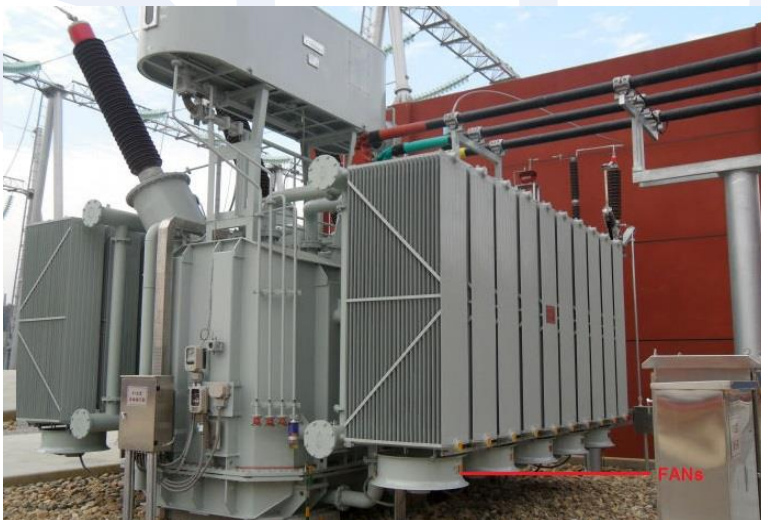
Fig (e): ONAF cooling of Transformer where fans are mounted below the radiators &
